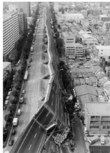
Fig. 1 Collapse of elevated bridges in 1995 Kobe earthquake
