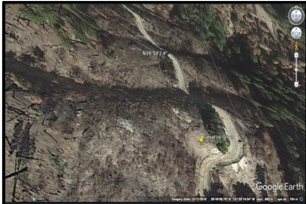
Fig. 4. Paradise Campfire Origins indicate downed power line towers. Were the tower bases melted? What forces destroyed the tower bases... simple wildfire propagation or strong ground solar induction currents? (Google Earth Image – 11 Dec. 2018)
