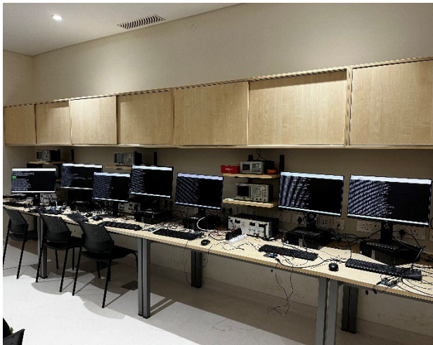
Figure 1. Actual cloudlet implementation using seven 410c
