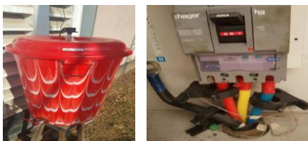
Figure 4: Sample Oil Sensor and Current Sensors Connection at Site
