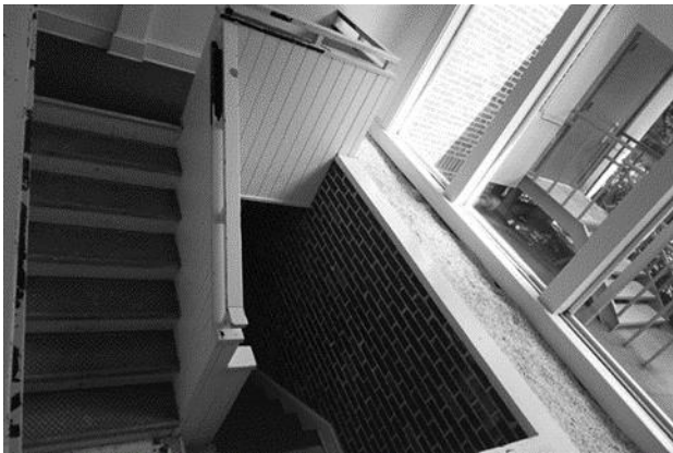
Fig. 4: Fine Arts Annex: stairway at main entry of 2nd/primary level; large glazing exposure at this stair creates both opportunities and challenges in the design scenario.
