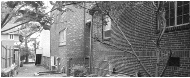
Fig. 3: Fine Arts Annex facing north: the tight confines along the western exposure with the neighboring property create a challenge when seeking to design a defensible zone around the building perimeter.
