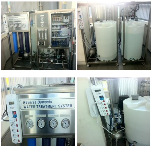
Figure 4. Measuring System Mounted in Small Size Desalination Plant
